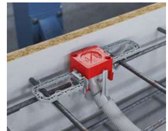
Prefix® upside mounting adapter (item no. 1261-00) - Easy and quick processing for installations above.
