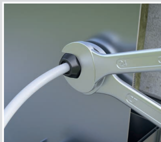
Pull the cable through and tighten the compression nut with a spanner
