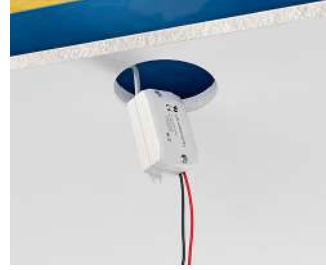
Installation of the operating device (driver).
