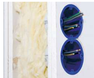
Use of a sound insulation box on one side of a double combination.
