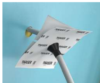
Remove the foil from the sleeve.
