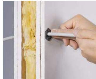
Press both sides of the sealing into each opening.
