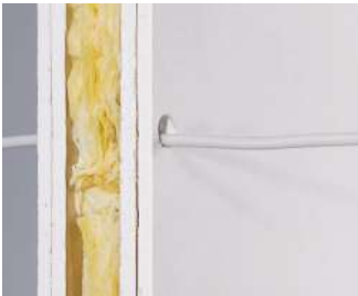
Cut an installation opening \varnothing 20 mm using a cutter (e.g. KAISER hardened metal cutter Art. No. 1088-06) or drill.
