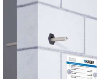
Wall feed-through in a sand-lime brick fire-protection wall.
