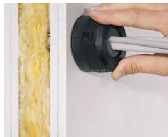
Place the sealing element on the seal cylinder and secure it with a 1/4-turn (bayonet fitting).
