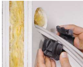
Place the two-part sealing cylinder around the cables and press together.
