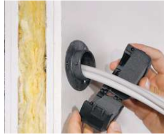
Open the sealing element and remove it.
