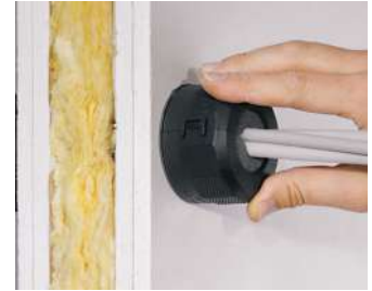
Place the sealing element around the cable, close it and secure it with a 1/4-turn clockwise.
