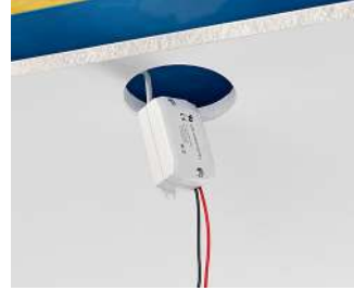
Installation of the operating device (driver).
