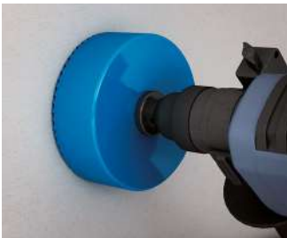
Cut installation opening with a cutter \varnothing 120 mm (e.g. bi-metal-cutter Art. No. 1082-20).
