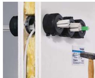
After installing the sealing, apply the identification tag.
