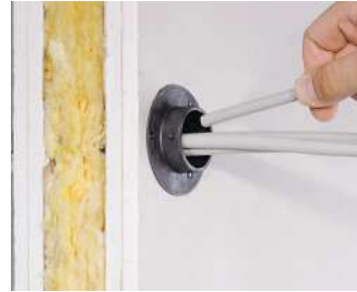
Insert the new cables.
