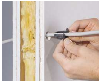
To install, open the sealing sideways and slide it over the cable.
