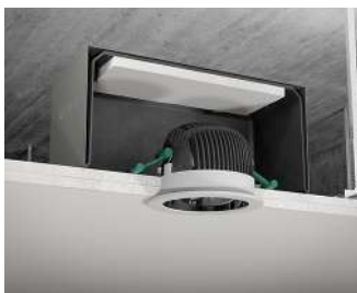
Fire-stop housing for recessed luminaires...
