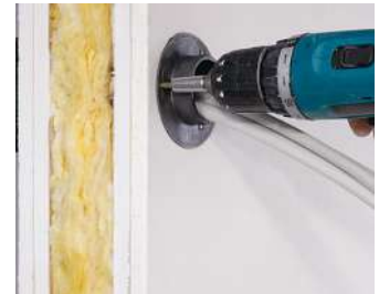
Fasten by tightening the screws (same procedure as for cavity wall boxes).
