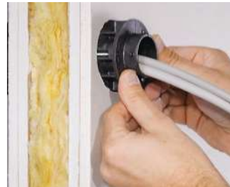
Press the sealing cylinder into the installation opening.
