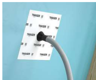
Stick on the sleeve and press firmly on to the base, working outwards from the centre.
