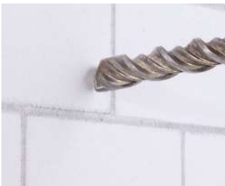
Make an installation opening using a Ø 32 mm drill.
